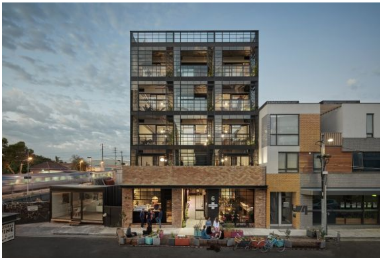
Breathe Architecture's Nightingale 1 took home the Allan and Beth Coldicutt Award for Sustainable Architecture. Image: Peter Clarke
