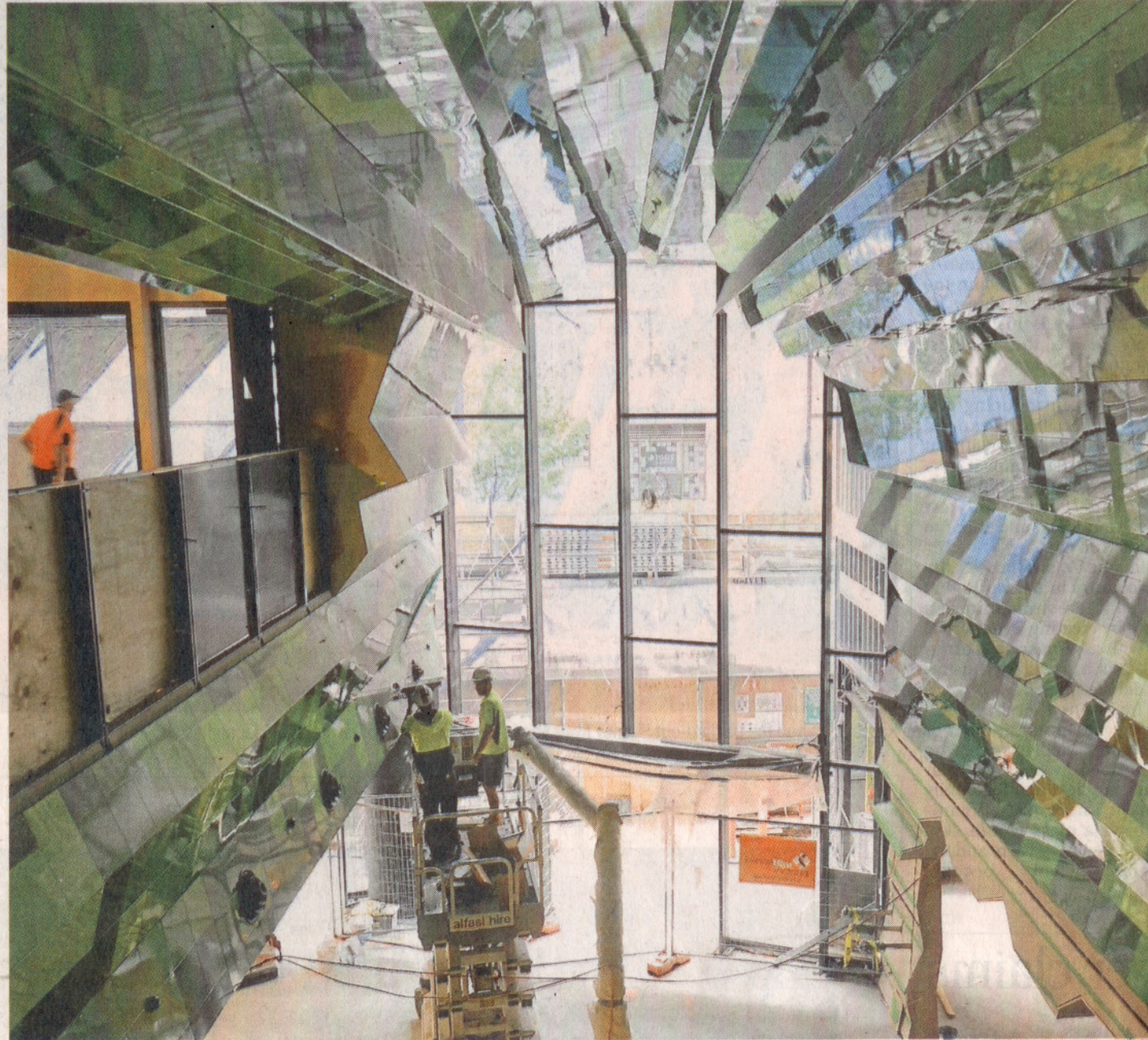
Construction workers are busy in RMIT's soon-to-be-completed Swanston Academic Building.
