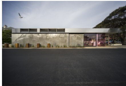
Sorrento Visitor Centre by Workshop Architecture. Image: John Gollings
